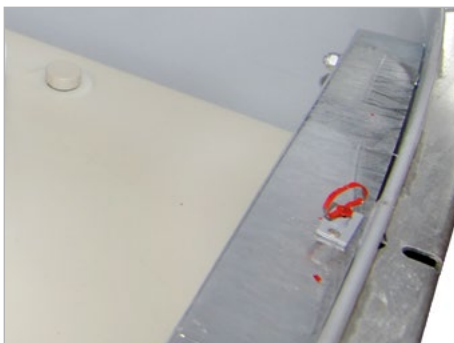
Dipstick to register any leakage
